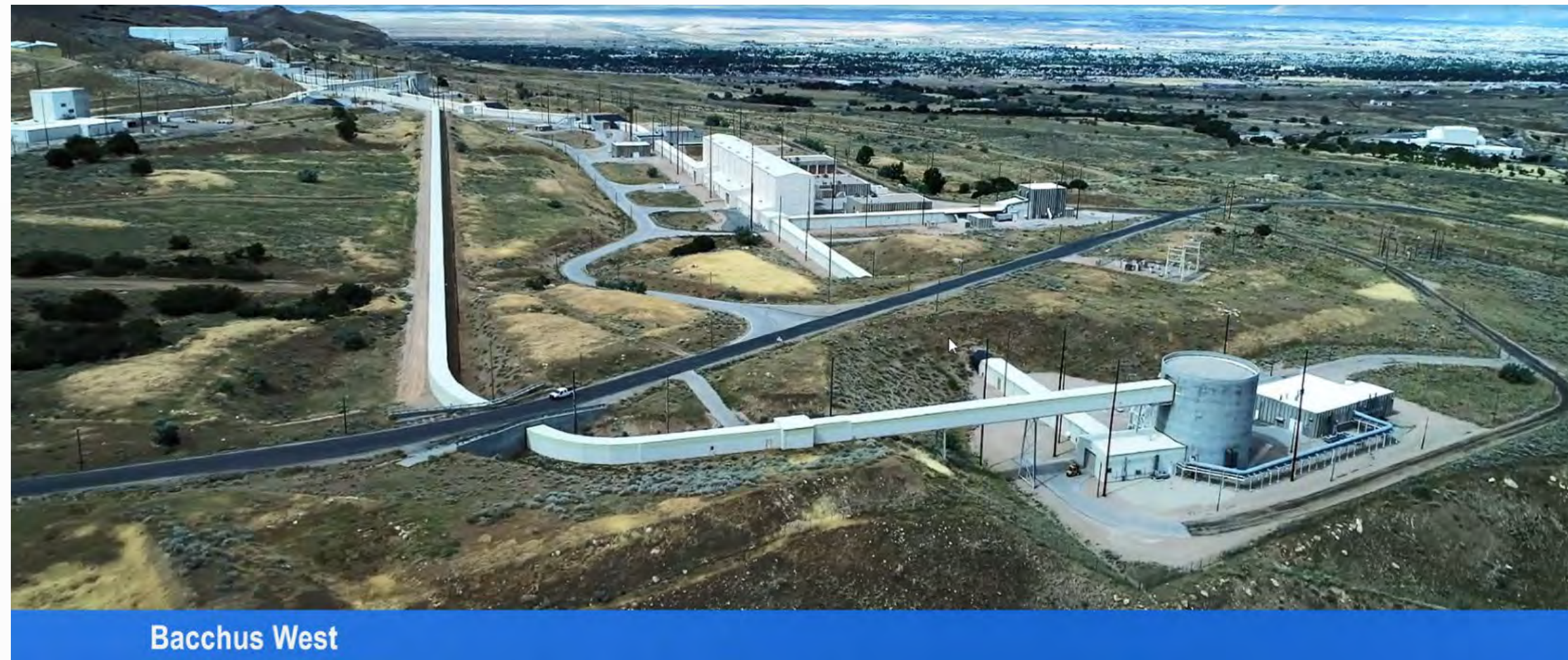
Figure 1. An aerial view of the NGC Bacchus West campus in Magna. The covered road is where the guide-by-wire system is used to direct the automated vehicles across the plant
