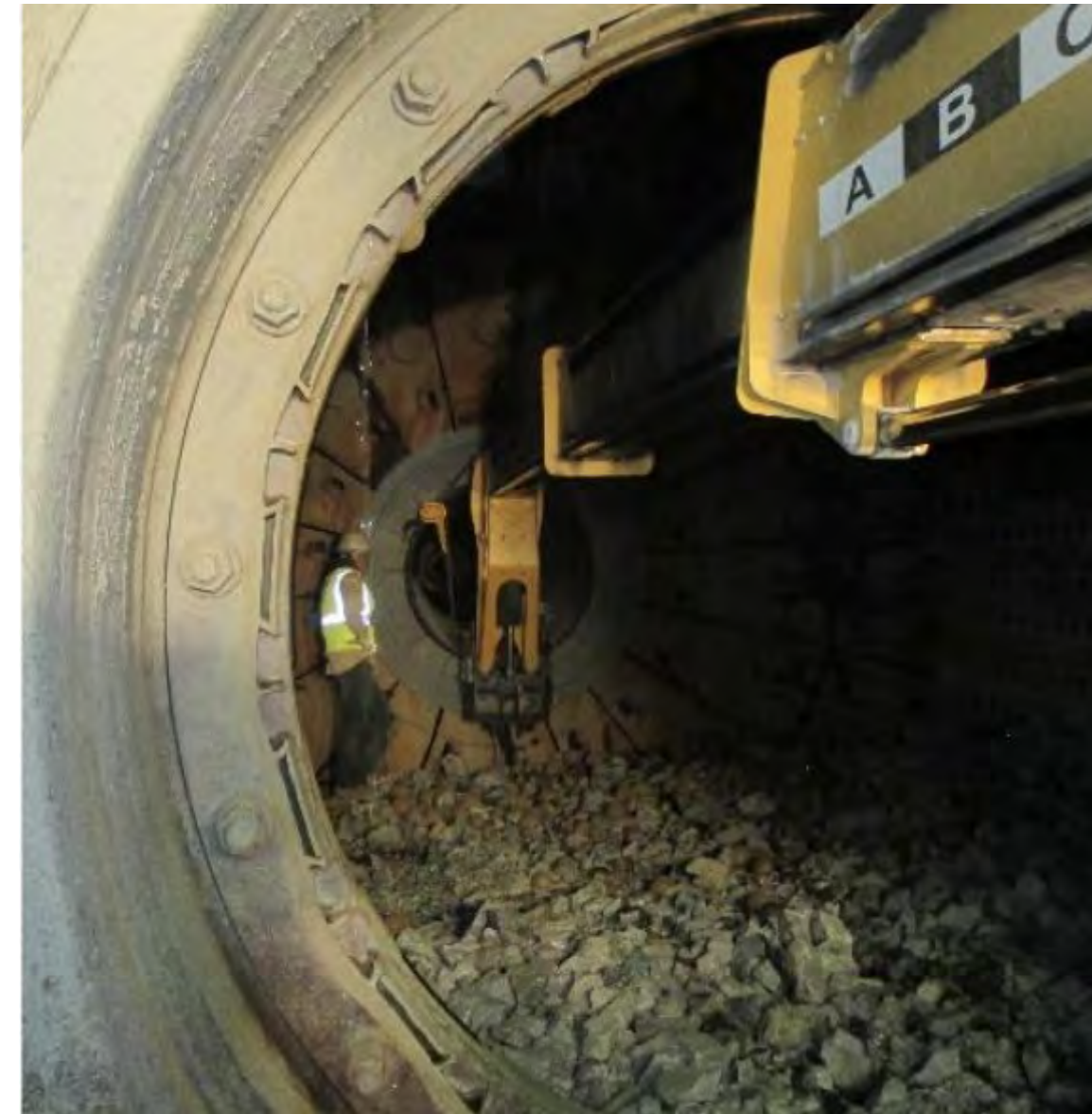
Fig 1: Example picture of current cone replacement process
